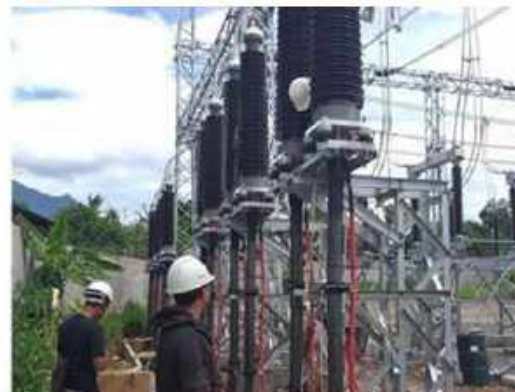
PEMASANGAN STEALING AND 150 KV
