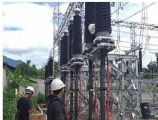
PEMASANGAN STEALING AND 150 KV
